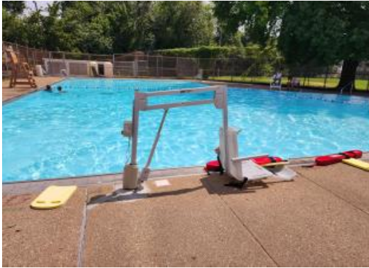
PHOTOGRAPH 7: VOGT POOL – While the chair lift can move up and down, it cannot swing from left to right, which prevents visitors from using it and lifeguards from properly and safely operating it.
