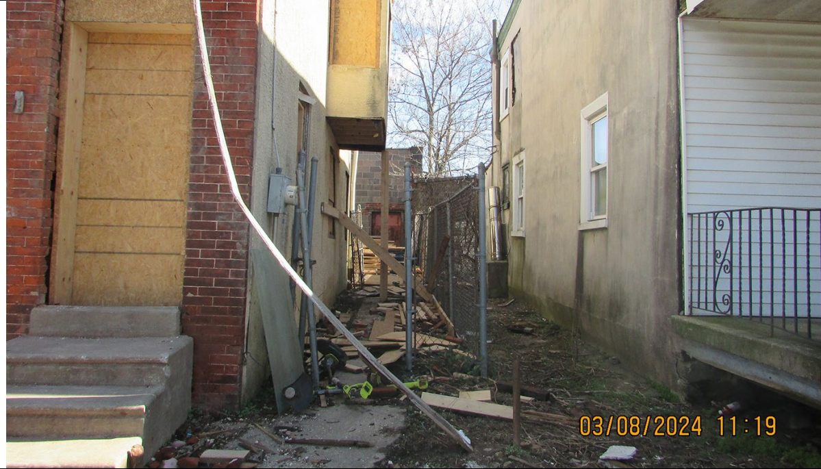
Supports were installed to maintain the ID property.
