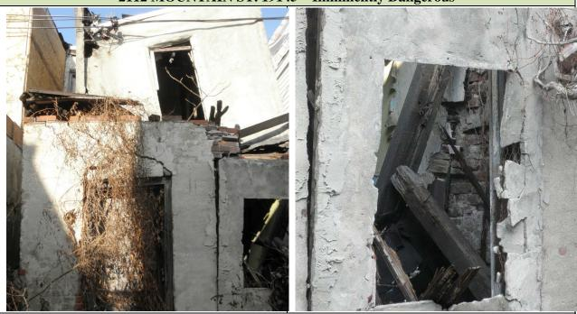
Last Inspection (Feb. 23, 2014): Rear of building is significantly damaged, as the top portion of it has collapsed into the lower level. L&I violations include wall, roof and floor partially collapsed.
