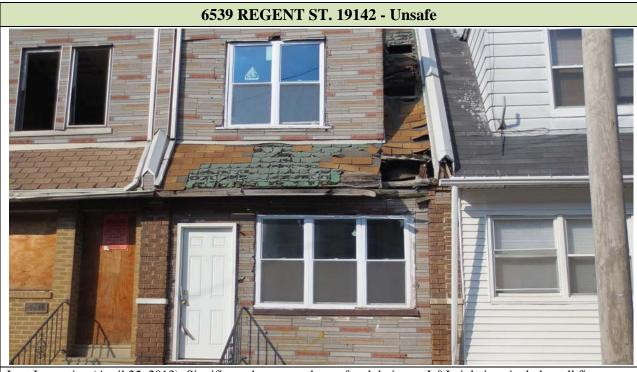
Last Inspection (April 25, 2013): Significant damage to the roof and drainage. L&I violations include wall fire damaged and the roof and wall deteriorated. Attached property had unsealed windows and No Trespassing sign.
