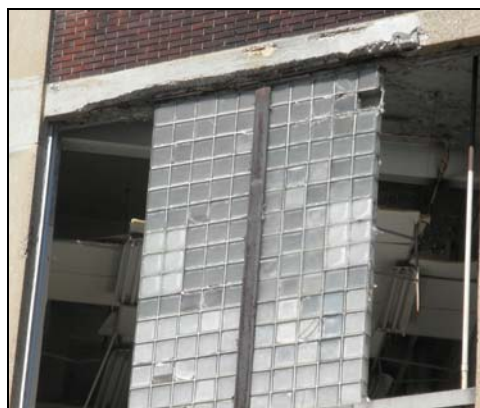
Missing windows and broken concrete, which has fallen to the ground, has weakened the overall structure of the former Roberto Clemente Middle School. It should be demolished immediately.
