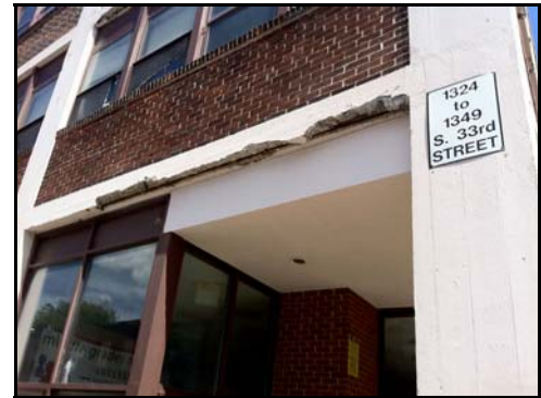
Exposed rebar and broken cement can be found around the entire building
