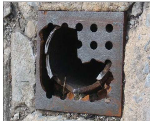
The open drain with the broken cover pictured above is a tripping hazard
