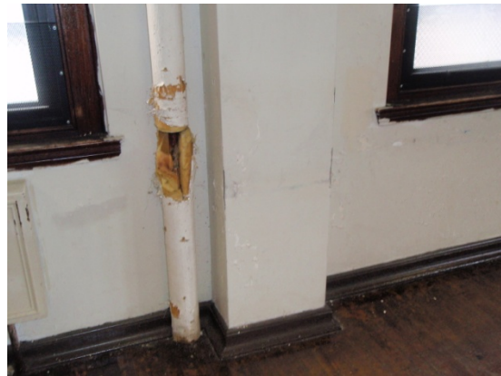
Figure 26 – Exposed Insulation – Dimner Beeber
