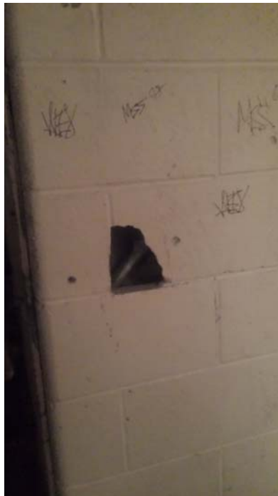
Damaged Masonry Wall: George Washington –Auditorium Backstage
