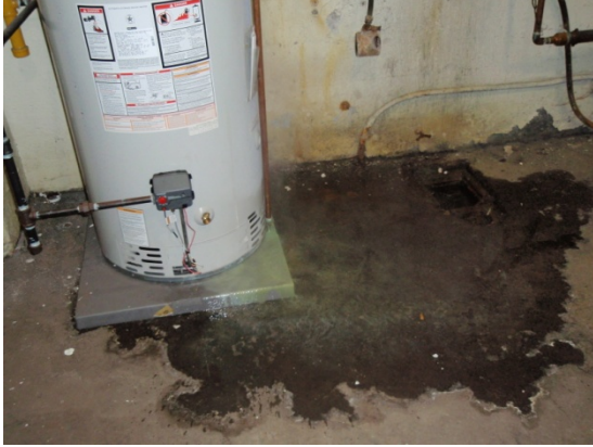
Figure 29 – Leaking Water Heater – Dimner Beeber
