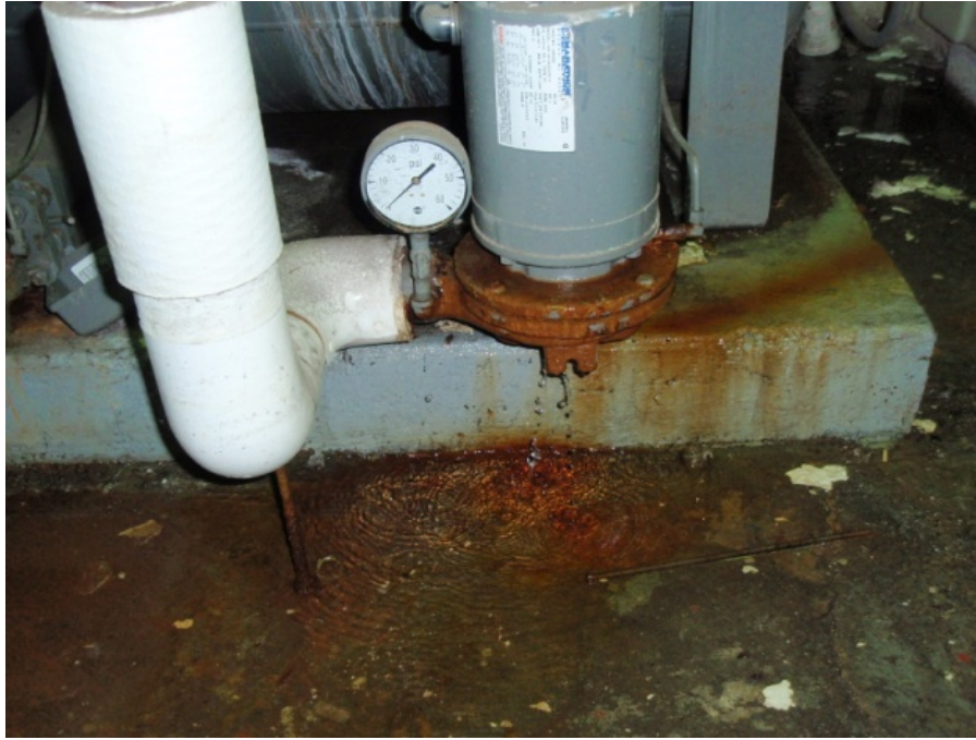
Leaking in the Mechanical Room: Dimner Beeber
