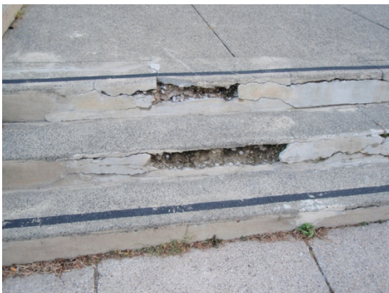
Figure 15 – Damaged Masonry Steps - Overbrook Education Center
