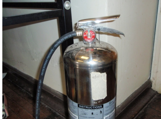
Figure 12 –Expired and Empty Fire Extinguisher – Dimner Beeber
