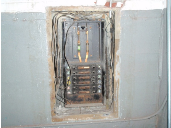
Figure 1 - Exposed Electrical Panel - Dimner Beeber
