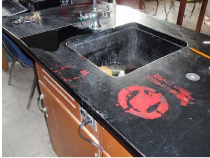
Outlet should have GFCI: Frankford High
