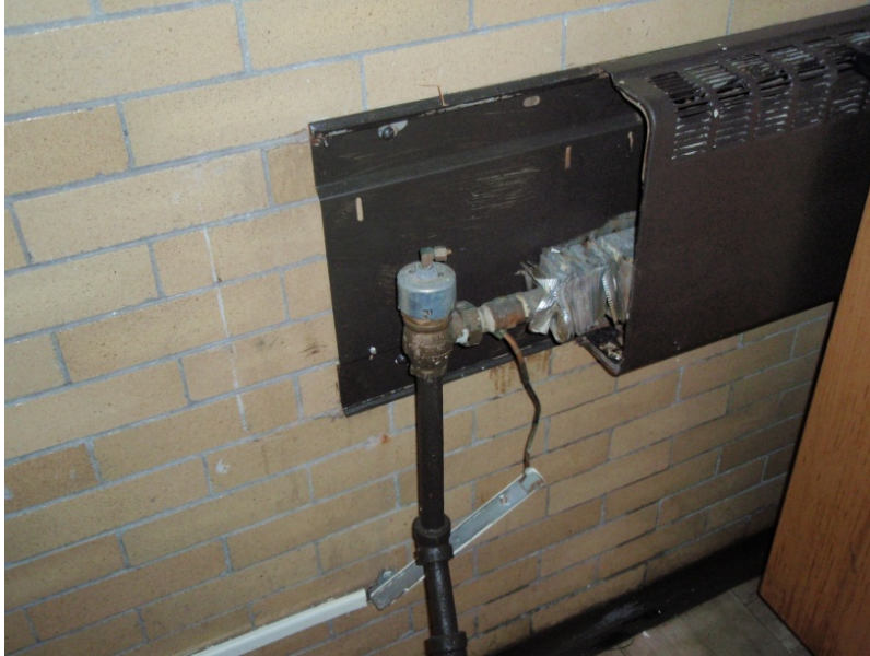
Damaged Heating System: Dimner Beeber
