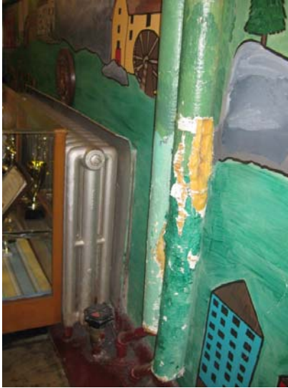
Exposed Insulation: John Story Jenks - Hallway
