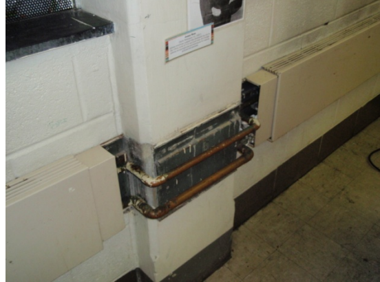
Figure 24 - Missing Heater Cover - Frankford
