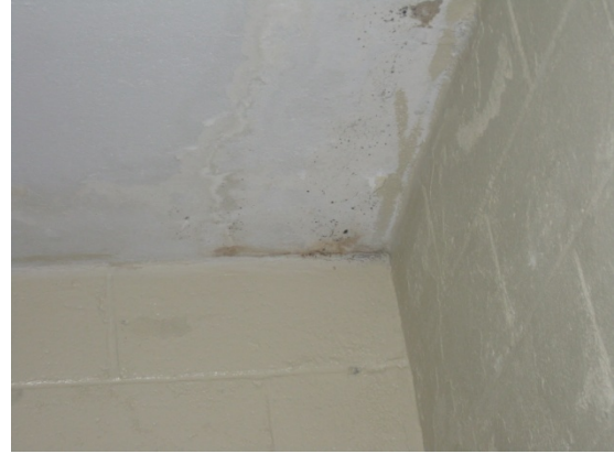
Figure 6 – Water Damage with Possible Mold – George Washington
