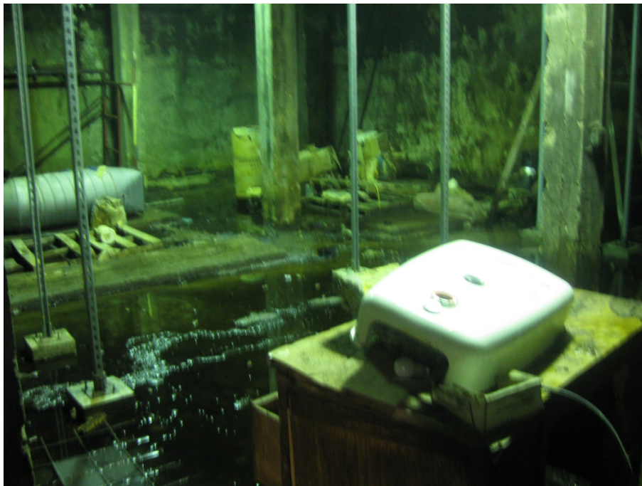
Leaking in the Mechanical Room: Kearny
