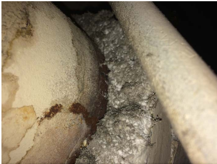
Asbestos insulation improperly terminated on a large pipe: Francis Scott Key - Hallway
