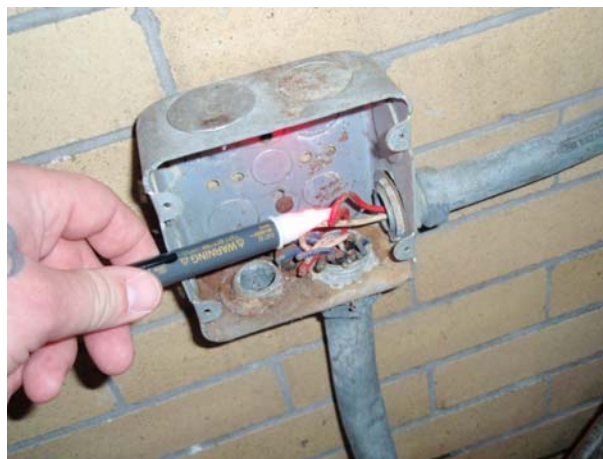
Exposed Wires: Dimner Beeber - Classroom
