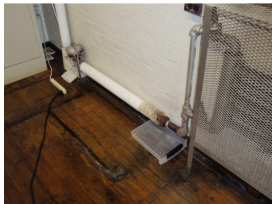
Figure 28 – Exposed Insulation and Leaking Heater – Francis Scott Key
