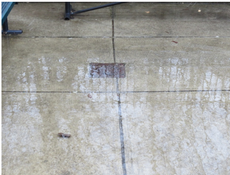
Clogged Storm Drain: Shawmont
