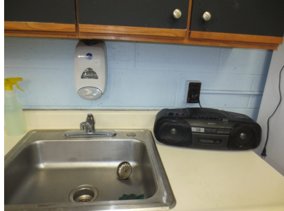
Figure 2 – Outlet next to a sink that should be a GFCI outlet – Cooke Wisahickon
