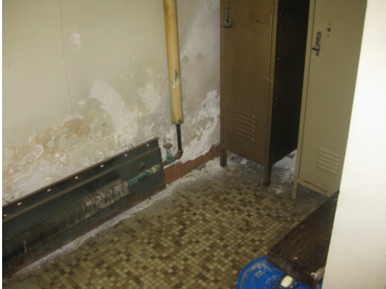
Figure 23 – Damaged Heating Unit – Bayard Taylor
