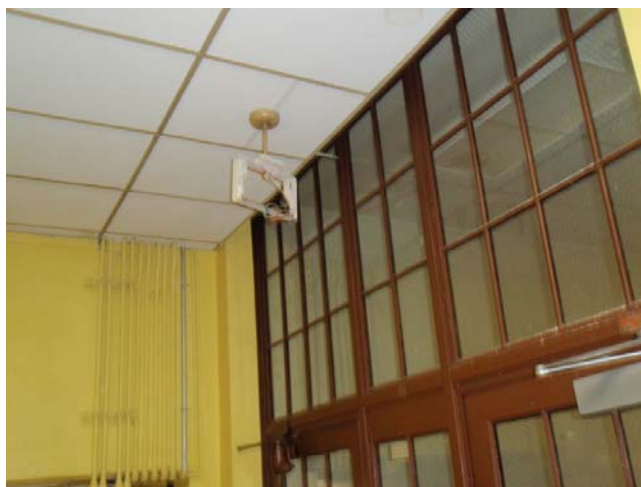
Damaged Fire Exit Sign: Martha Washington
