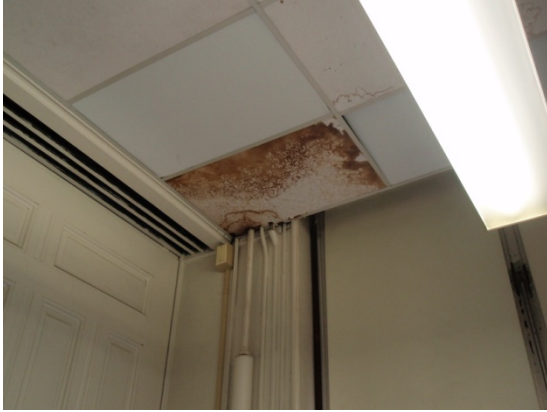
Figure 5 – Water Damage – Francis Scott Key
