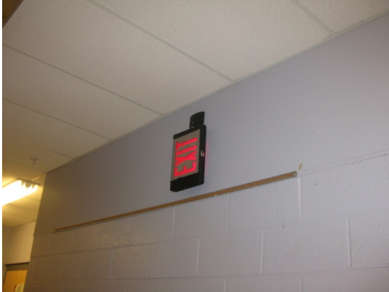
Figure 11 – Damaged Fire Exit Sign – Juniata Park
