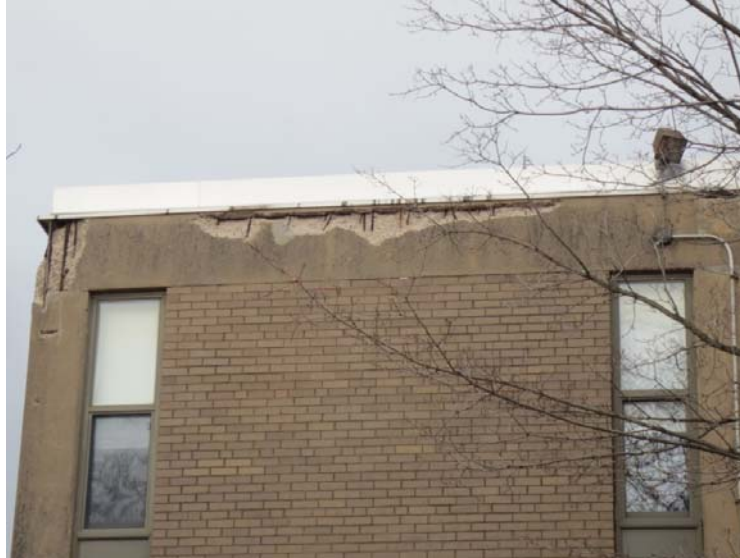
Damaged Masonry: Cooke Wisahickon
