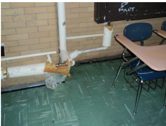
Figure 27 – Exposed Insulation – Dimner Beeber
