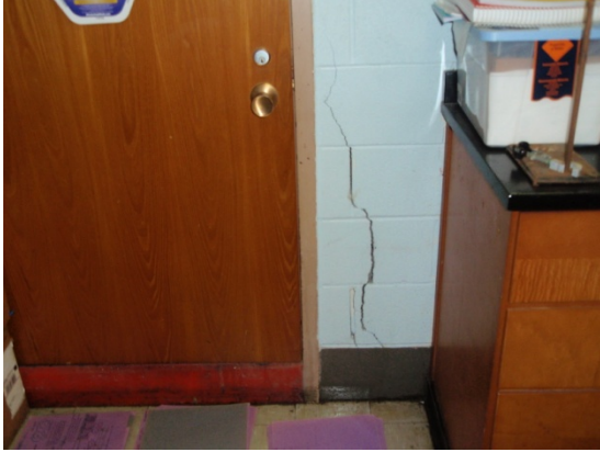
Figure 17 – Damaged Masonry Wall - Frankford
