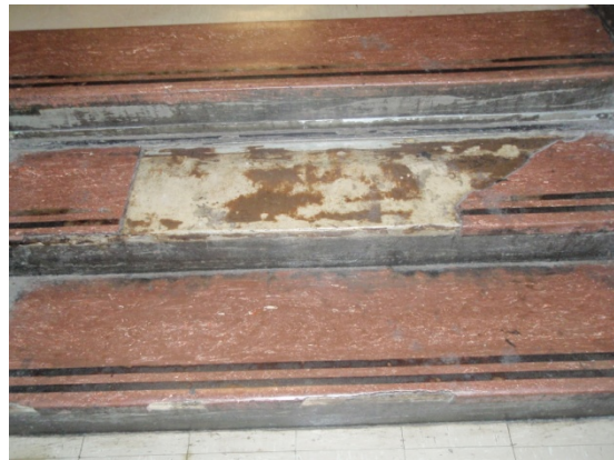
Figure 14 – Tripping Hazard, Damaged Step - Frankford
