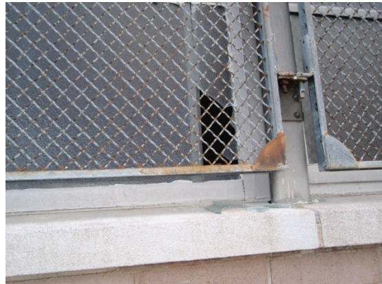
Figure 20 – Broken Window – Martha Washington
