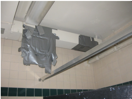
Figure 31 – Damaged Air Duct – John Story Jenks
