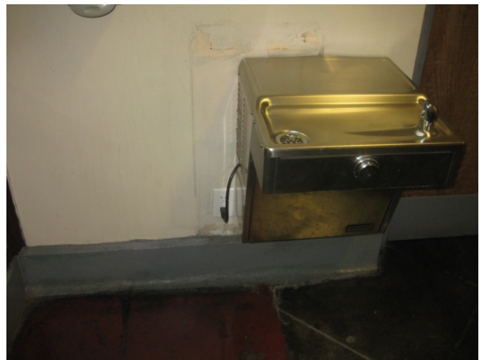
Bayard Taylor Elementary School – Before - Water fountain missing a GFCI outlet. After - GFCI outlet installed.
