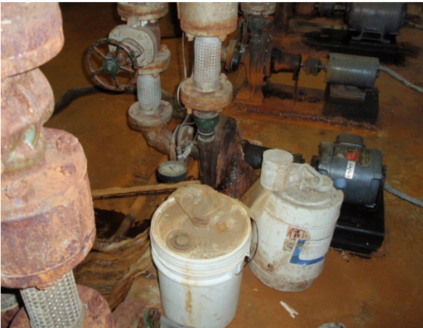
Frankford High - Before - Heating System circulator pumps leaking and bad bearings. After - All new circulating pumps and isolation valves installed on the heating system.
