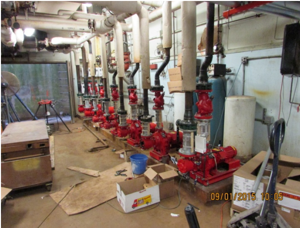
Frankford High - Before - Heating System circulator pumps leaking and bad bearings. After - All new circulating pumps and isolation valves installed on the heating system.
