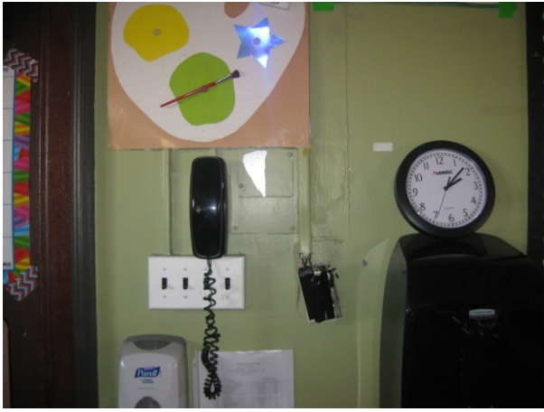
Andrew Jackson Elementary School – Before - Damaged outlet with exposed wires. After - Repaired outlet and wires.
