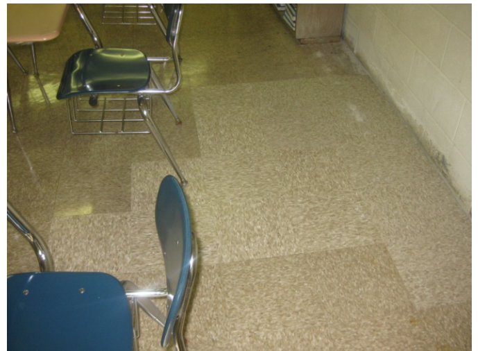
George Washington High School – Before - Damaged tile floor. After - Floor repaired.
