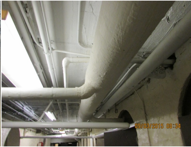
Francis Scott Key Elementary - Before - Asbestos wrapping in bad shape. After - Asbestos insulation encapsulated, properly sealed, plaster ceiling repaired and freshly painted.
