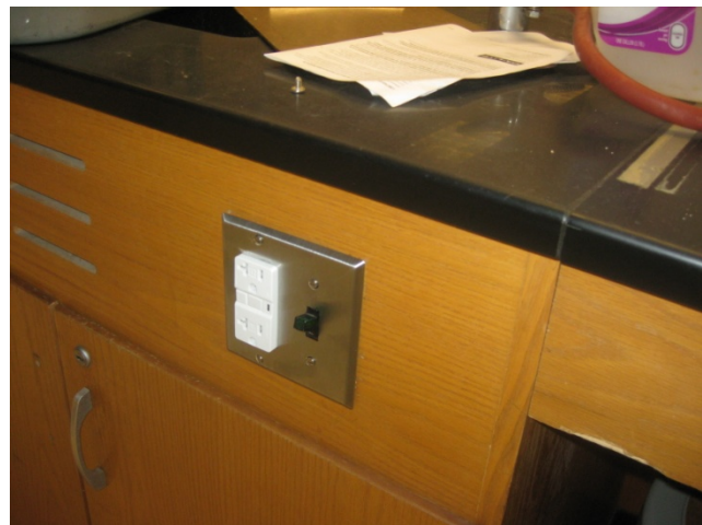
Central High School – Before - Outlet near a water source without a GFCI outlet. After - GFCI outlet installed.
