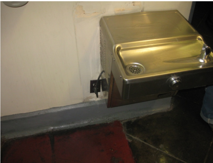
Bayard Taylor Elementary School – Before - Water fountain missing a GFCI outlet. After - GFCI outlet installed.
