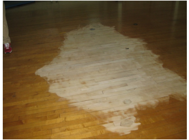
George Washington High School – Before - Buckled floor. After - Floor repaired.
