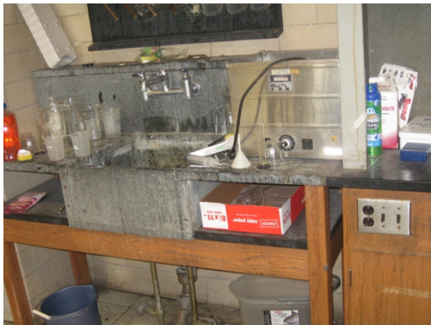
Central High School – Before - Outlet near a water source without a GFCI outlet. After - GFCI outlet installed.
