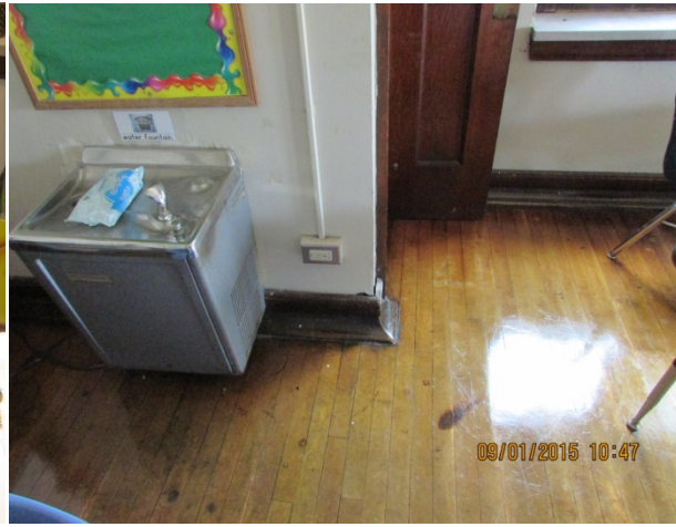
Crossan Elementary - Before - No GFCI next to a water fountain. After - New GFCI's installed throughout.
