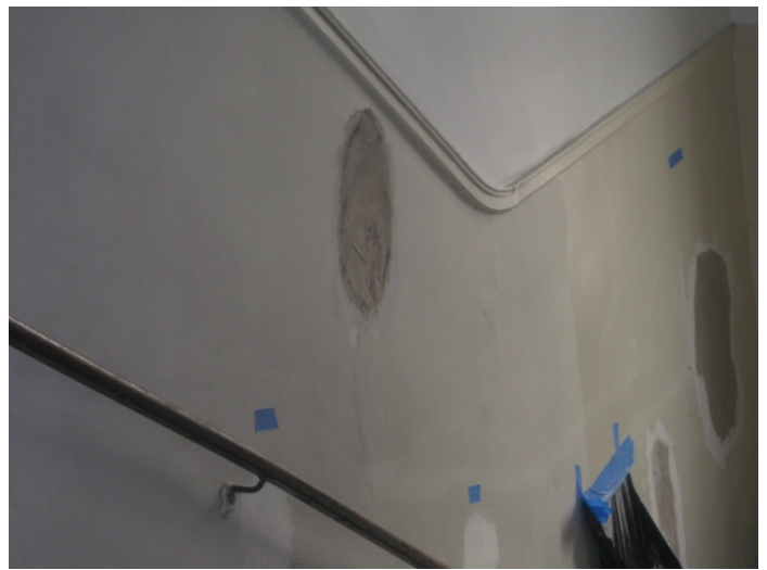
Bayard Taylor Elementary School – Before - Damaged plaster. After - Plaster work in progress.
