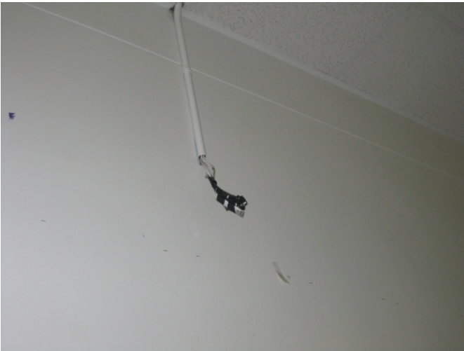
Bayard Taylor Elementary School – Before - Wires were improperly terminated. After - Wires are capped.
