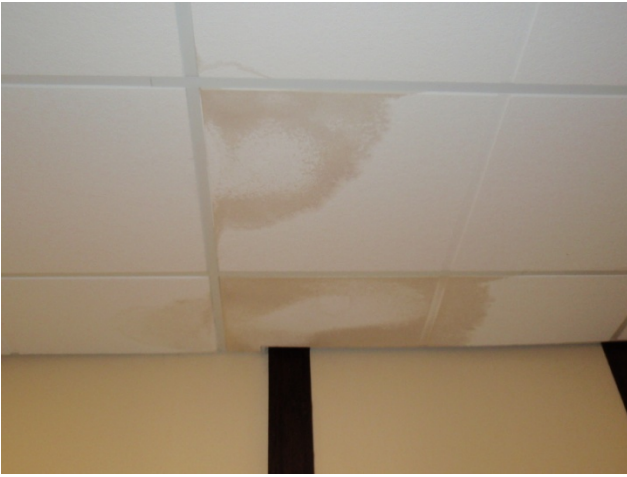
Delaplaine McDaniel Elementary School – Before - damaged ceiling tiles. After – Tiles were replaced.
