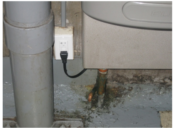
General Kearny Elementary School - Before - Water fountain without a GFCI outlet. After - GFCI outlet installed.
