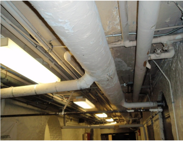
Francis Scott Key Elementary - Before - Asbestos wrapping in bad shape. After - Asbestos insulation encapsulated, properly sealed, plaster ceiling repaired and freshly painted.
