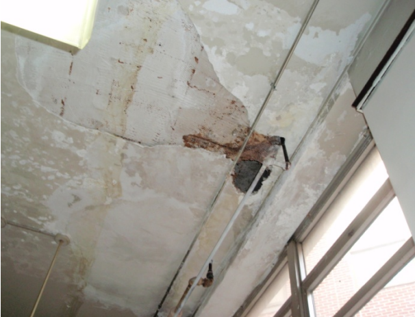
Frankford High - Before - Severely Damaged Plaster 2nd Floor Hallway. After - New plaster repairs and fresh paint throughout the school.
