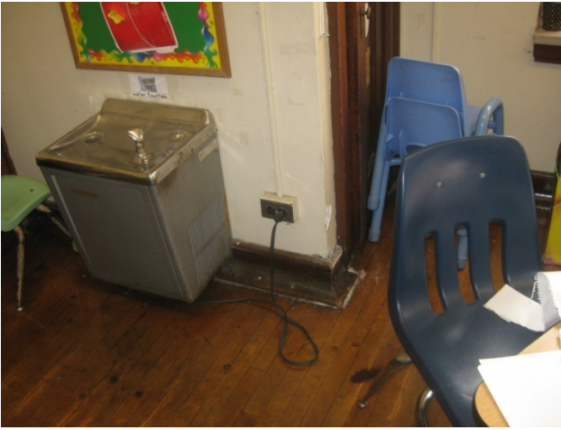
Crossan Elementary - Before - No GFCI next to a water fountain. After - New GFCI's installed throughout.
