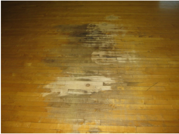
George Washington High School – Before - Buckled floor. After - Floor repaired.
