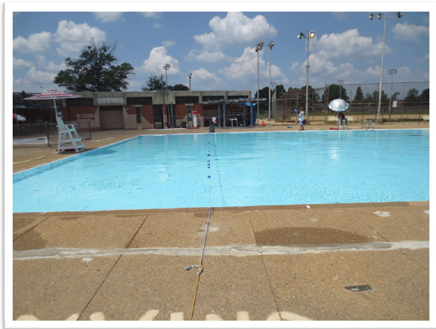
Safety lines tied across pool and deck areas – Tripping Hazard
