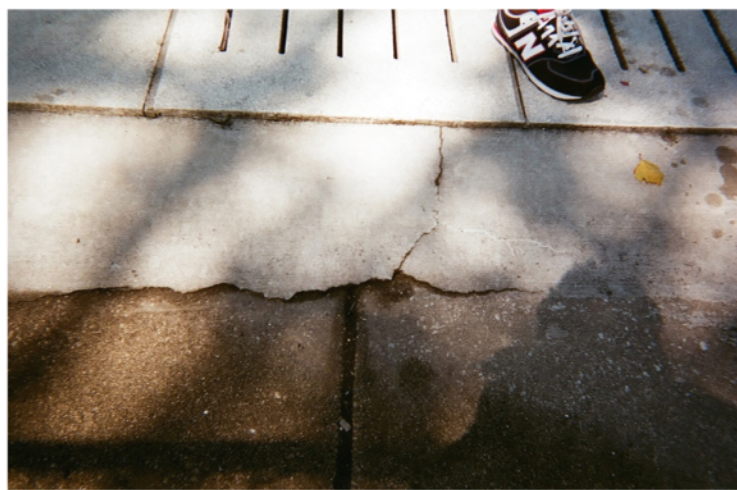
Mill Creek Pool Un-even Surface Tripping Hazard
