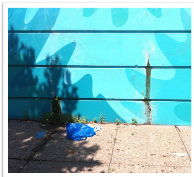
48 th & Woodland Avenue Sprayground Leaking water through wall from defective drainpipe from sprayground area
