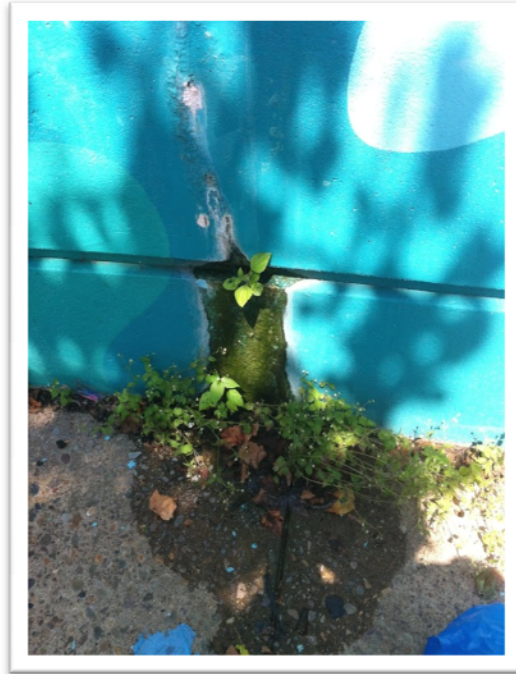
48 th & Woodland Avenue Sprayground Broken drain pipe from sprayground leaking through wall onto Woodland Avenue pavement
