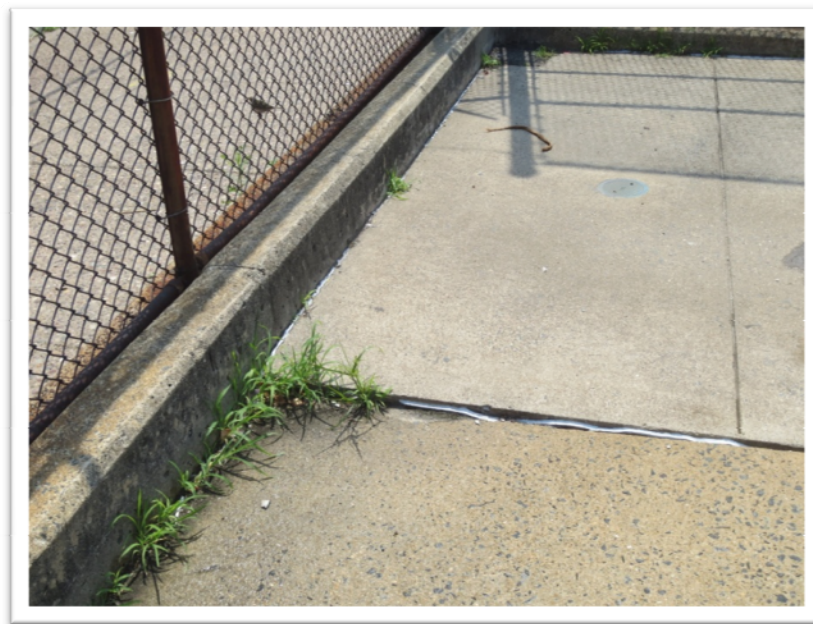
East Poplar Pool – Un-Even Concrete Pool Area Tripping Hazard
