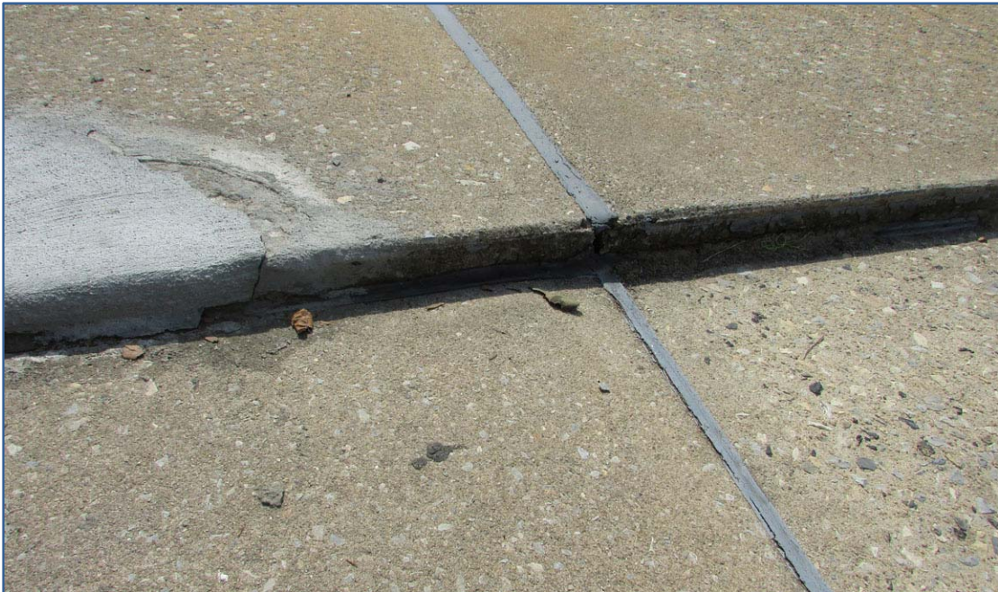
Stinger Square – Uneven Pavement, Tripping Hazard
