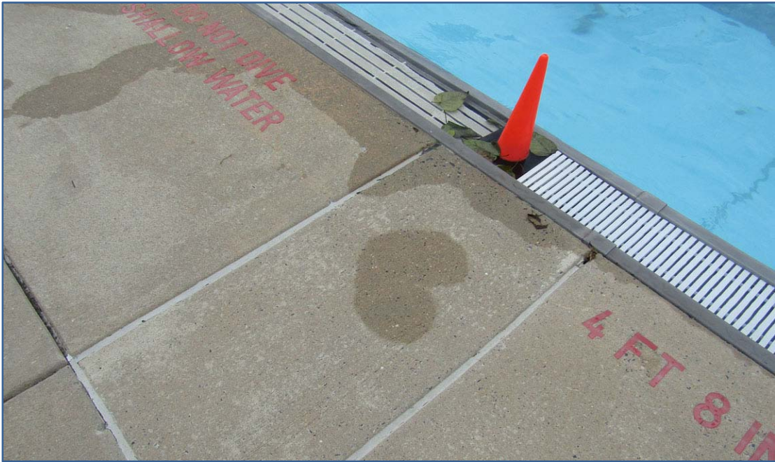
Stinger Square – Uneven Pavement, Tripping Hazard
