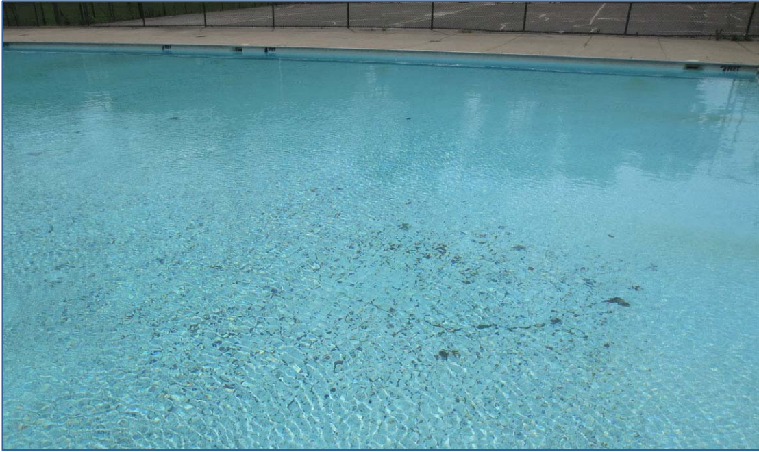
Belfield Pool – Paint Peeling
