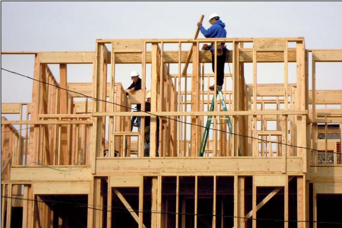
Figure 5 – Worker is standing on the top rung of step ladder. (site 5)
