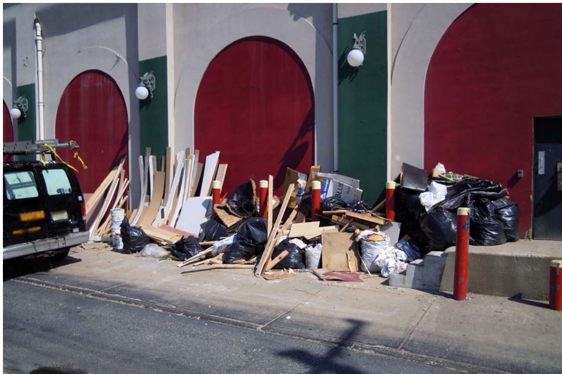
Figure 14 – Debris blocking egress path. (site 15)
