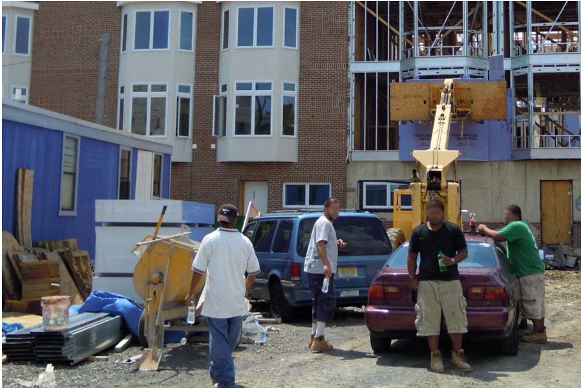
Figure 1 – Workers stated they were being paid cash. (site 21)
