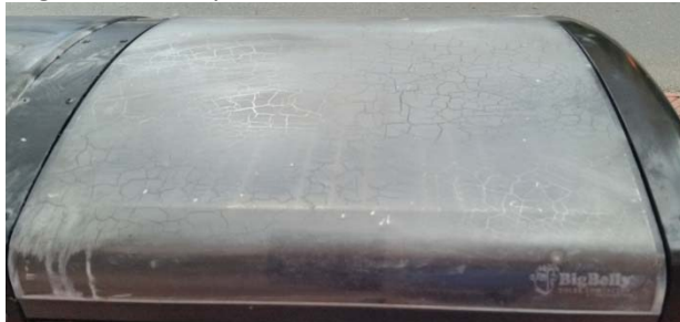
Solar Bubble severely weathered, 4 th & Market NW, August 12, 2016
