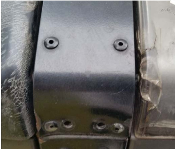
7 th & Arch NW, Cracked Solar Bubble and missing screws and rear panel damaged, September 20, 2016
