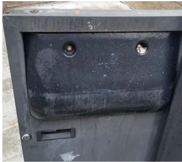
Door Handle Missing, 12 th & Locust, July 18, 2016
