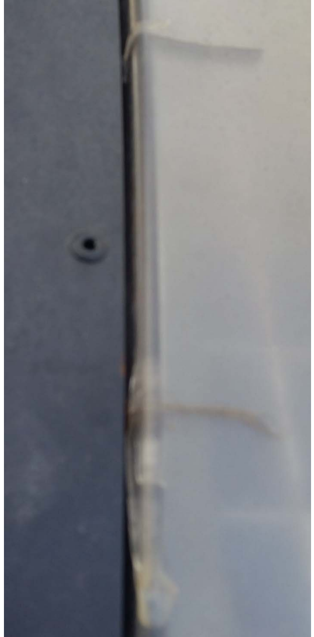
Solar Bubble cracked in numerous places, 7 th & Arch, August 8, 2016
