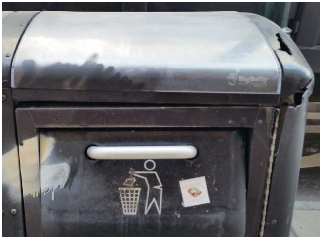
Severe damage, door not properly aligned, 12 th & Chestnut, February 15, 2017
