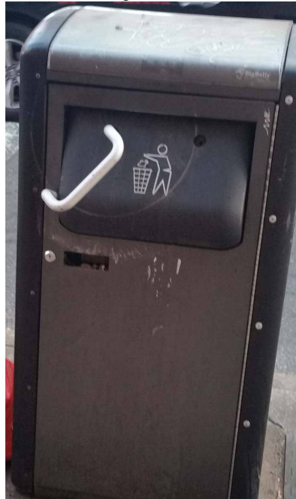
Handle broken, 10 th & Race, February 6, 2017 Also noted on March 24, April 18 and May 31, 2017 This item was also noted by Streets Dept crew and supervisor on April 21, 2017 but, as of May 31, had not been repaired.
