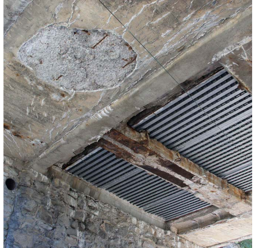
AFTER (2013) – Spalled concrete continues on encased beams, more steel has become exposed since 2009
