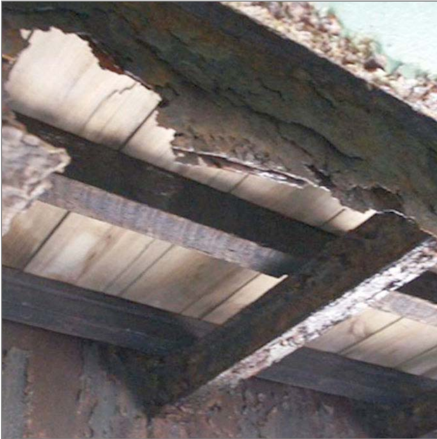
Significant corrosion of steel beams under the bridge, weakening the overall structure
