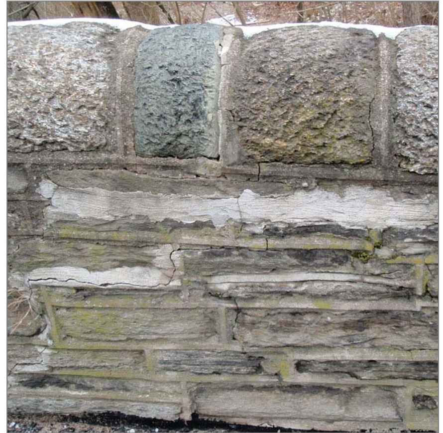
Cracking in the side wall of the bridge resulting in on-going damage
