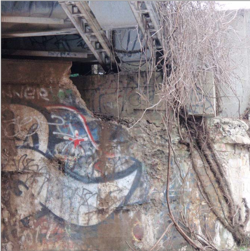
Significant amount of concrete missing under the bridge support
