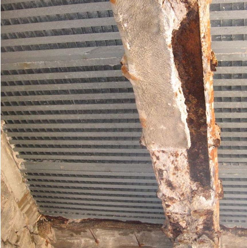
BEFORE (2009) – Spalled concrete on concrete encased beams, steel is corroded
