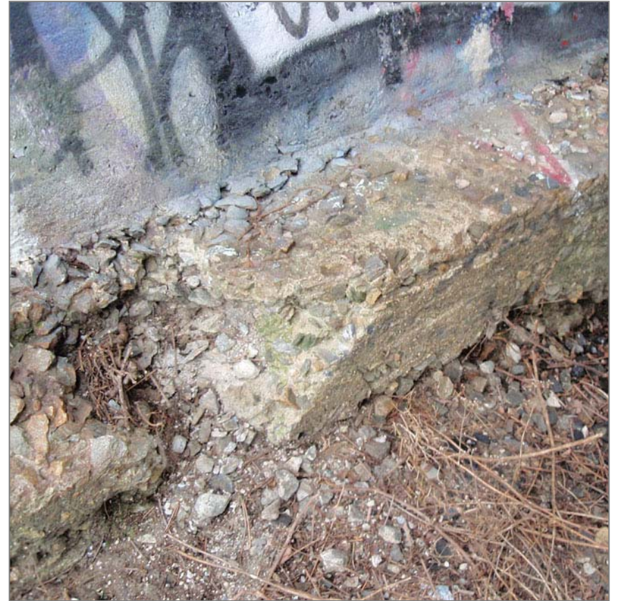
Concrete base damaged and missing sections of cement
