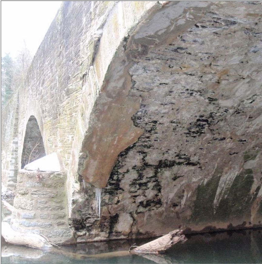
Concrete falling from the underside of the bridge weakening the overall support
