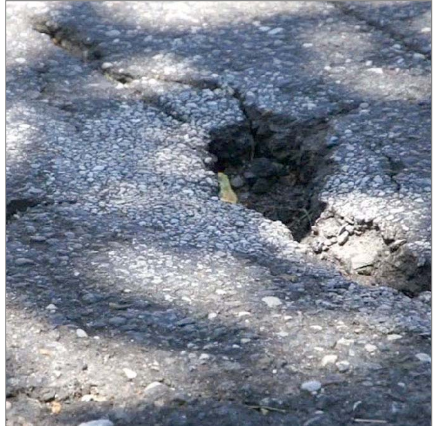
Pothole created by ongoing surface damage across the bridge
