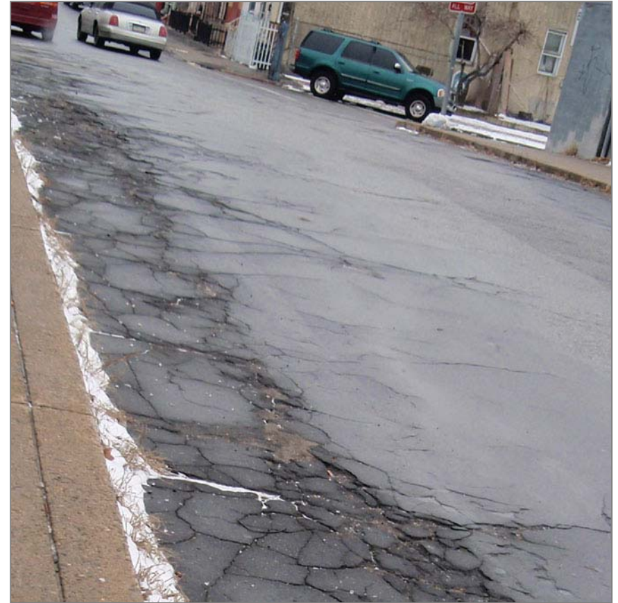
Surface cracking, known as Alligator Cracking, is present across the bridge. Ongoing cracking that goes unrepaired results in additional future costs
