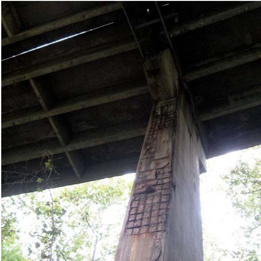
BEFORE (2009) – Concrete spalling with exposed rebar on pier
