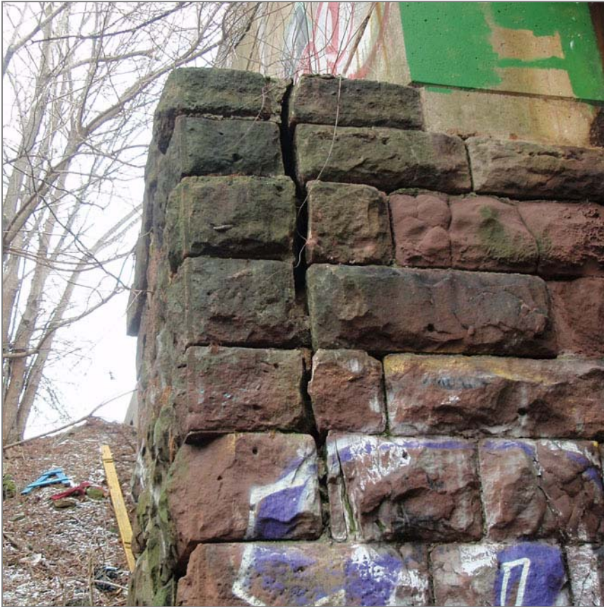
Large crack in the cement support under the bridge
