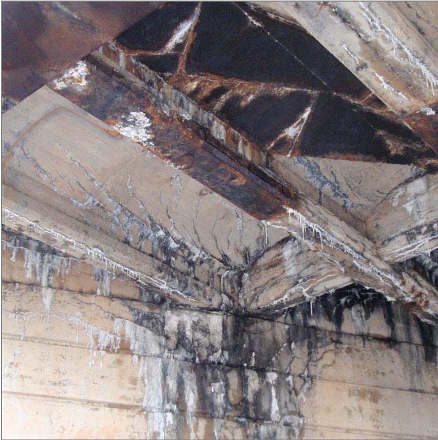
Steel plates under the bridge that are rusting and slowly deteriorating the structure
