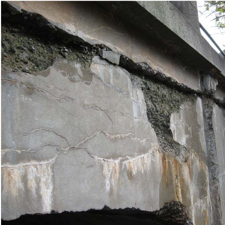
BEFORE (2009) – Concrete spalling on each side of the bridge
