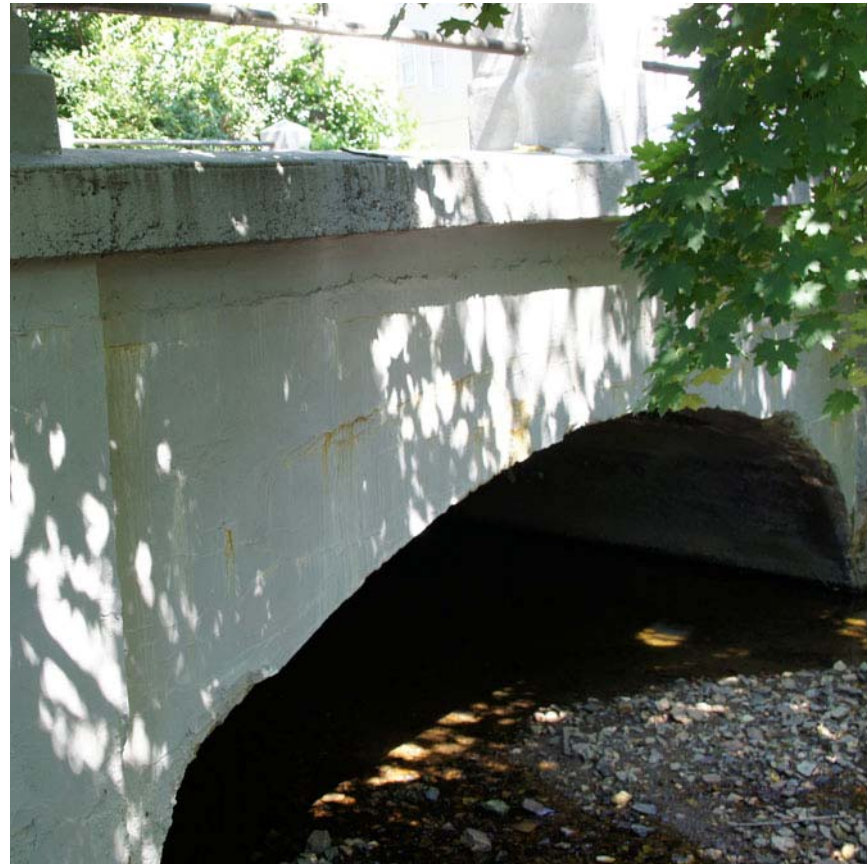
AFTER (2013) – Concrete has been replaced and it is no longer spalling
