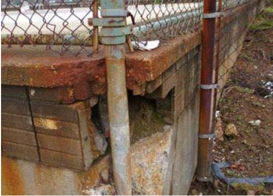
Figure 1 Broken Concrete: Amos
