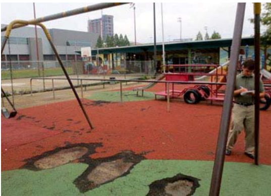
Figure 3 – Missing Swings and Damaged Safety Mat: Amos
