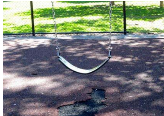
Figure 82 – Damaged Safety Surface: Wharton
