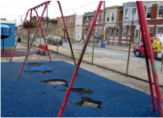
Figure 79 – Damaged Safety Surface and Missing Swings: Stokley
