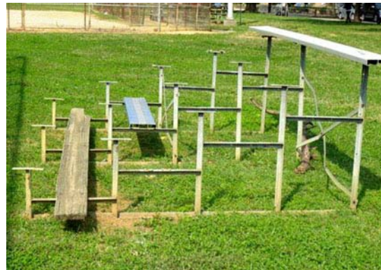
Figure 36 – Damaged Bleachers: Lawncrest
