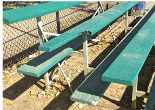
Figure 18 – Damaged Bleachers: Columbus
