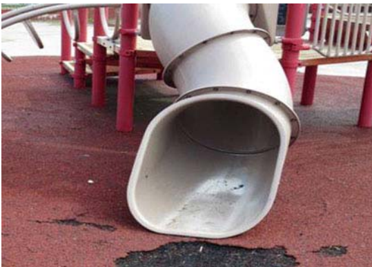
Figure 83 – Damaged Safety Surface: Ziehler
