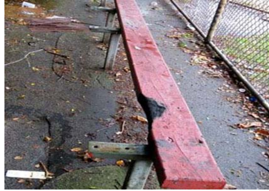
Figure 26 - Broken Bench: Heitzman
