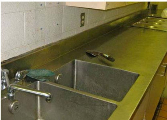
Figure 11 – Outlet should have GFCI: Carousel House
