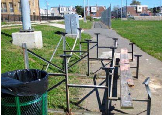
Figure 49 – Damaged Bleacher: McCreech
