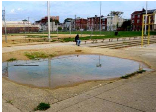
Clogged Storm Drain: Cruz
