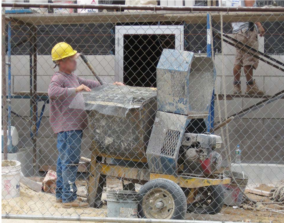
Picture 7. Missing dust screens
