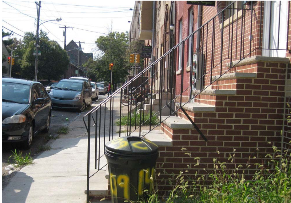
Picture 2. Stairs properly directed to the side to reduce encroachment on the sidewalk
