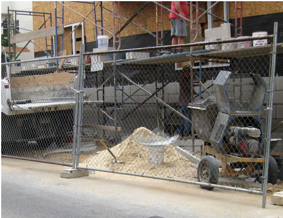
Picture 6. Lack of properly maintained silt fence or compost filter tube
