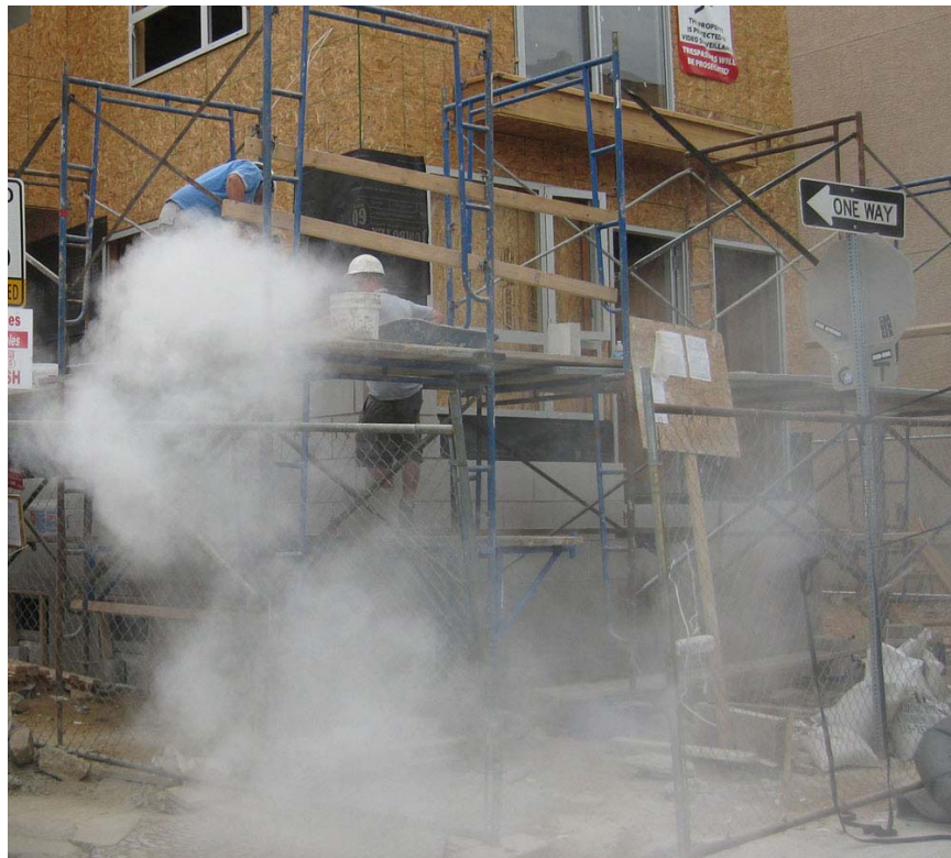
Picture 4. Air vacuum hose not being used on a saw to collect dust
