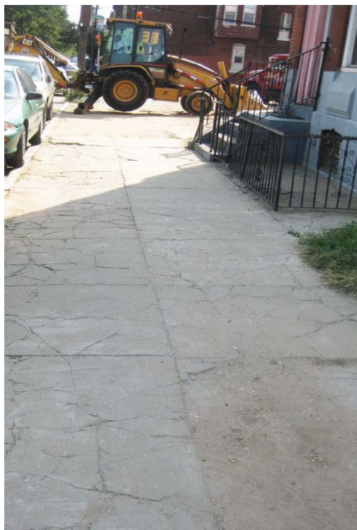
Picture 14. Sidewalk cracked likely due to construction trucks and heavy equipment parking on it.
