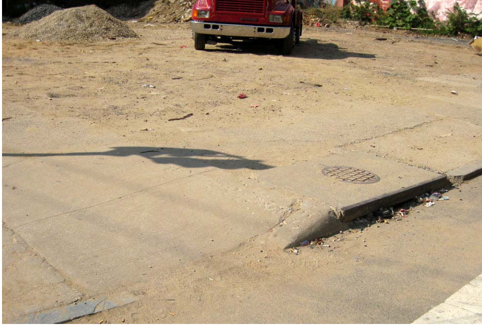
Picture 3. Lack of proper stormwater inlet protection
