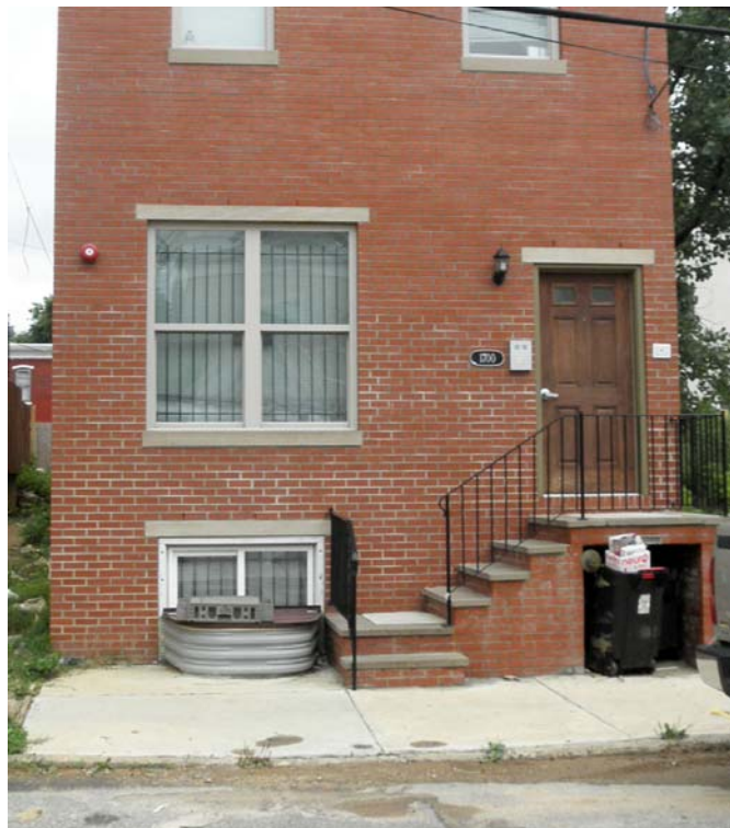
Picture 2. Stairs properly directed to the side to reduce encroachment on the sidewalk
